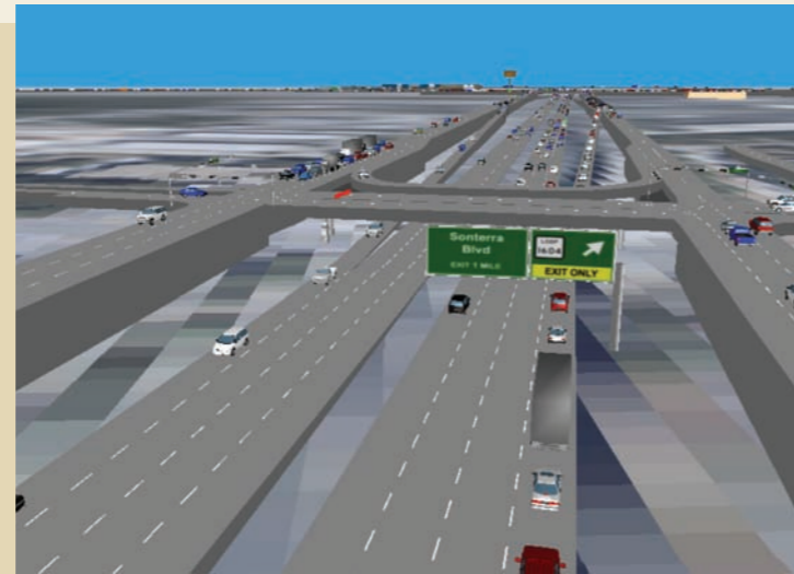
EXISTING NB US 281 AT EXIT TO LOOP 1604
