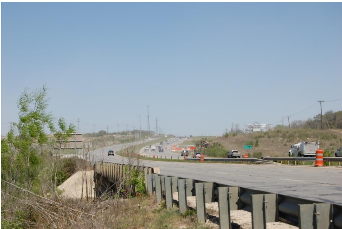
US 281 approaching Loop 1604, view facing north
