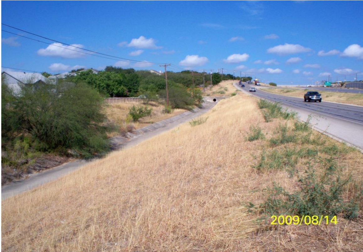
1604 Right-of-way, view facing west at Mudd Creek
