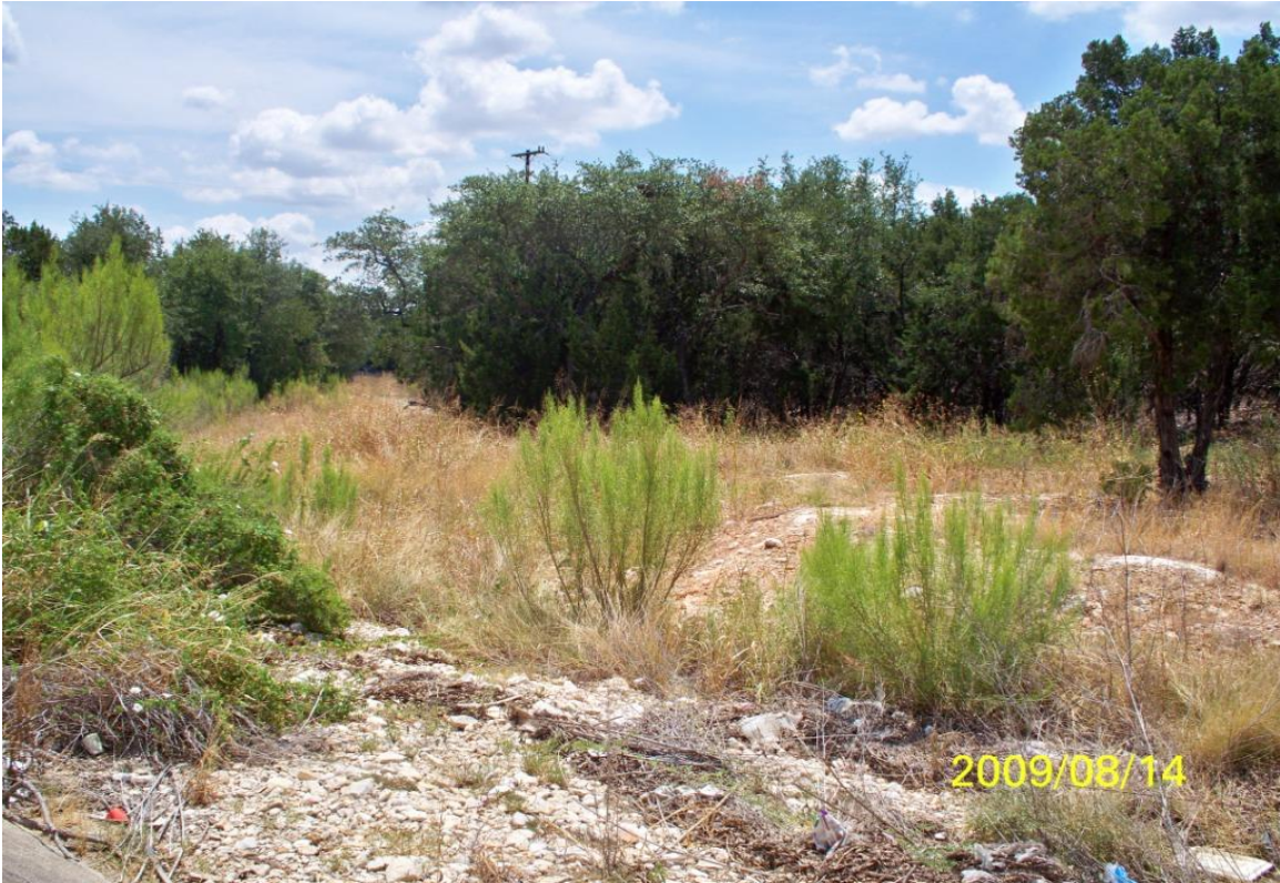
Facing downstream from large RCPs, south of Loop 1604
