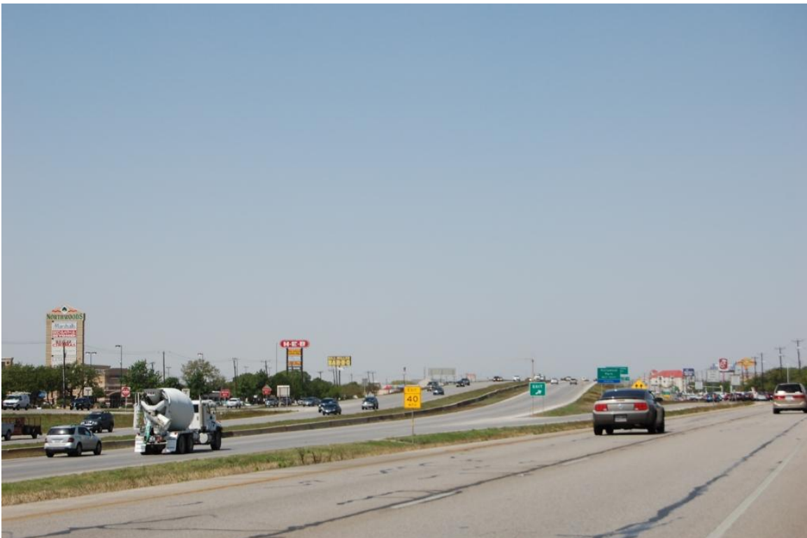
Loop 1604 approaching US 281; view facing west
