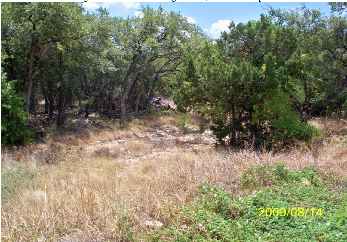
Facing south of culverts between Bitters and Huebner
