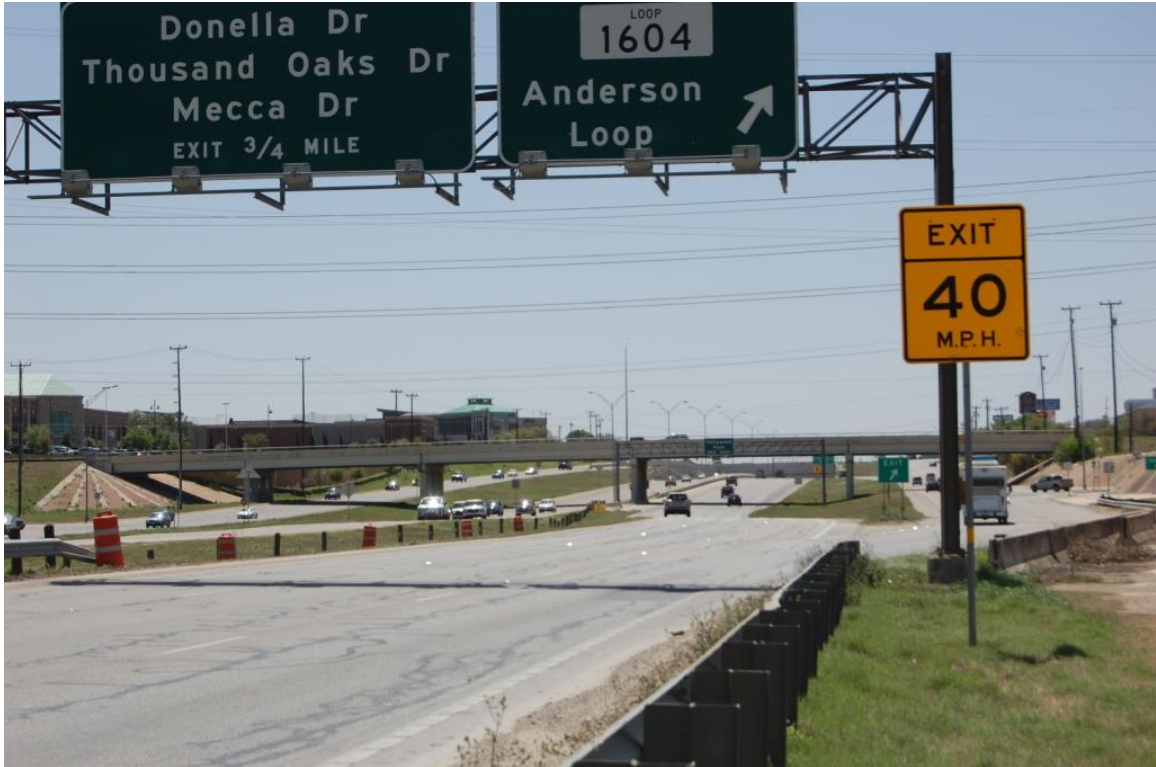
US 281, view facing south
